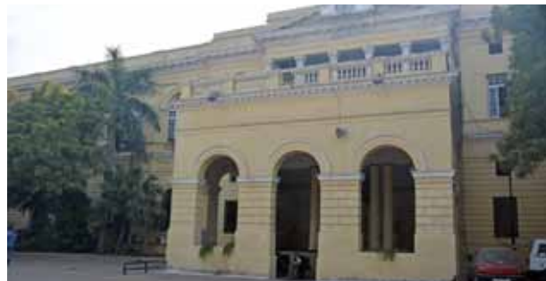
Inside the Town Hall premises
